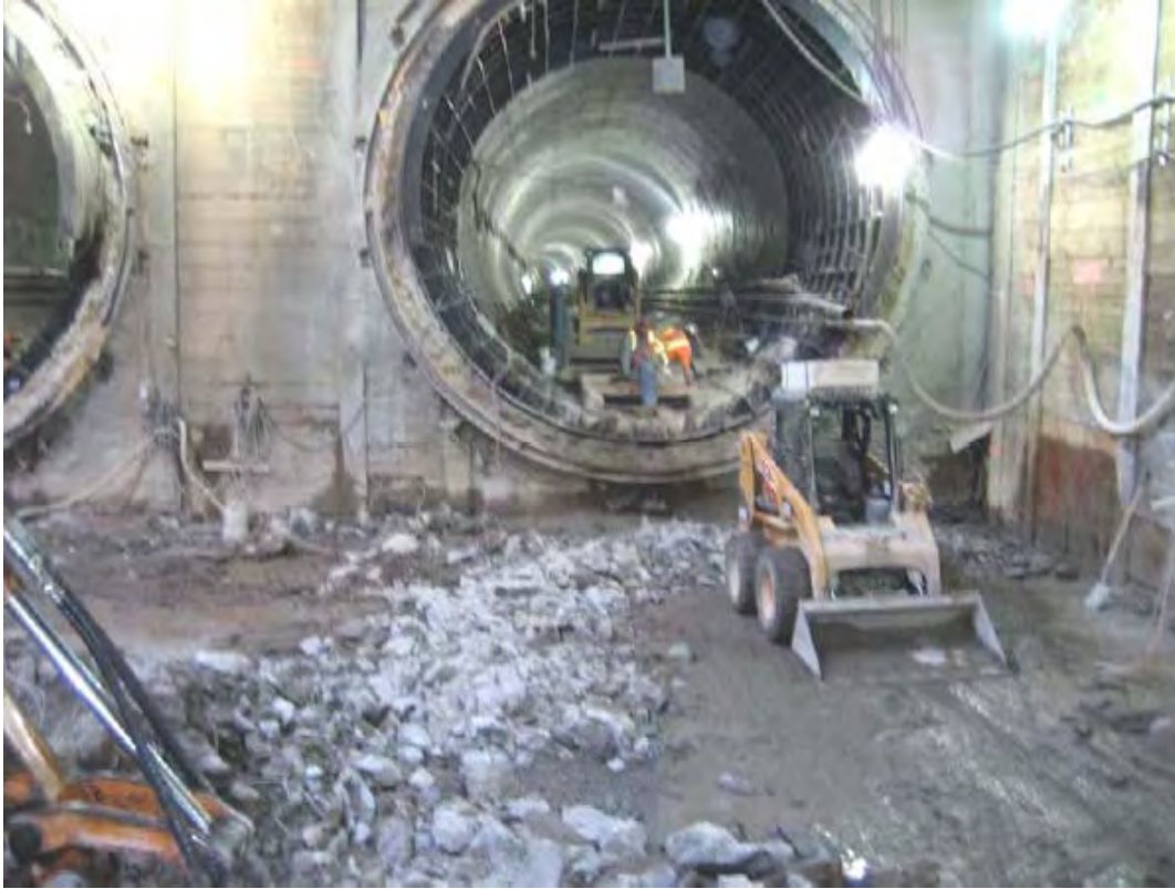
Gold Line Eastside Extension Project – West End of Soto Station
