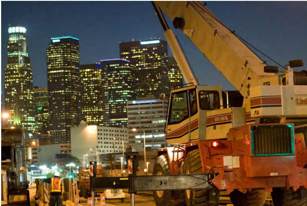
Gold Line Eastside Extension – Laying Track along First Street
