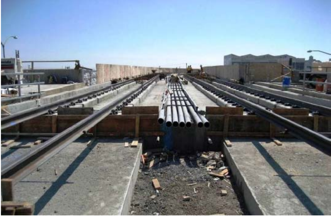
Guideway Construction on the US 101 Freeway Bridge Overcrossing
