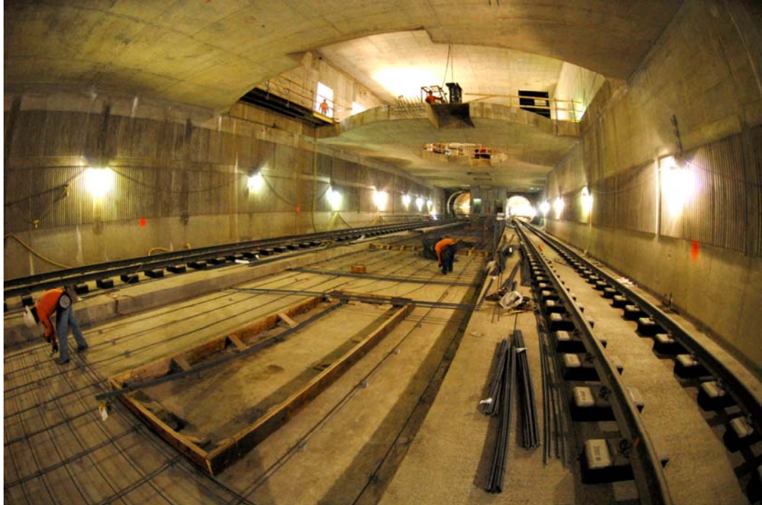
Soto Station Construction
