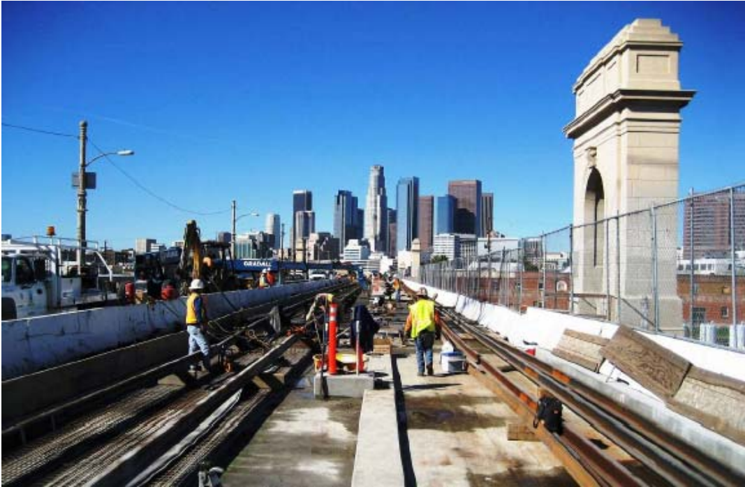
1st Street Bridge Construction
