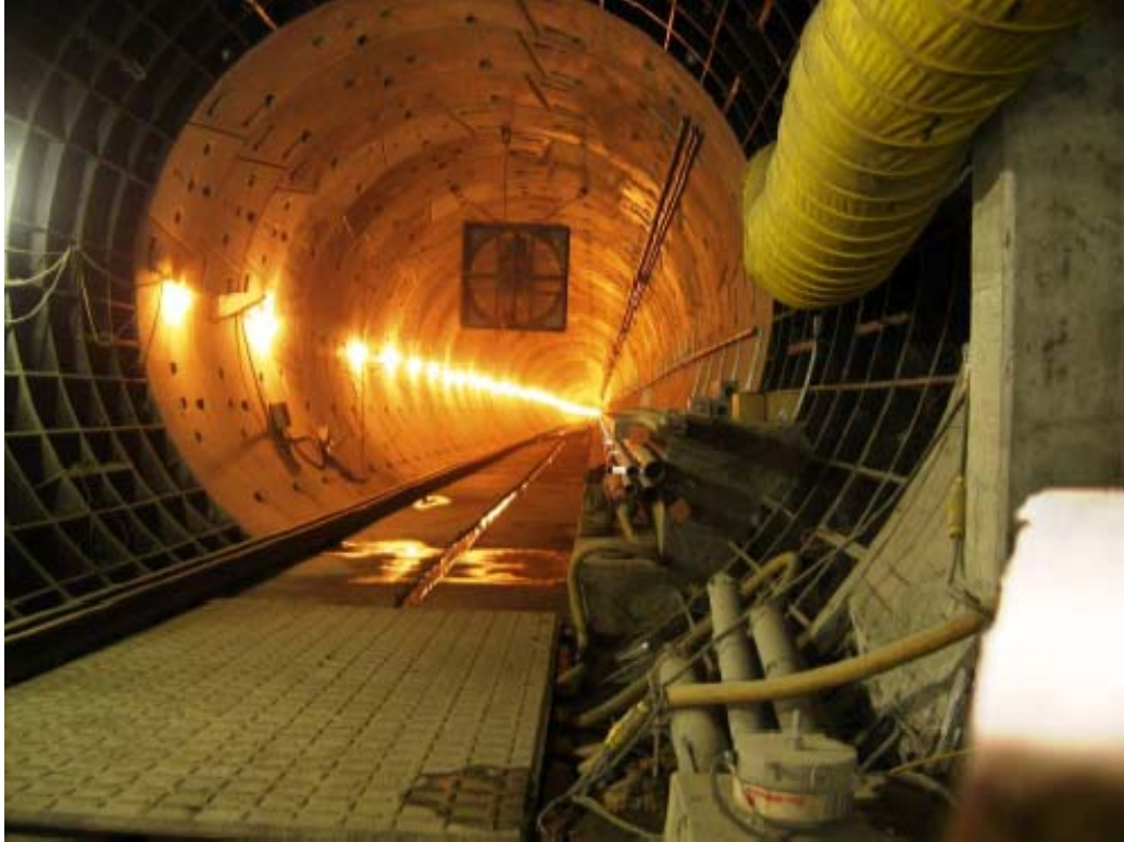
Westbound Tunnel Looking East of Soto Station
