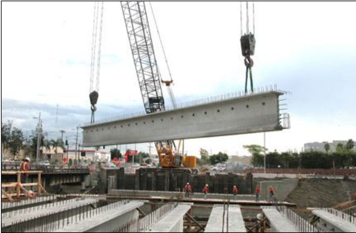
Installation of Girders for National Bridge
